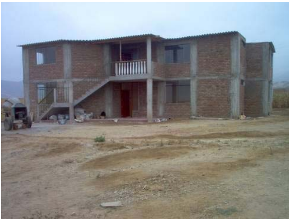
The Children's rooms are finished, just small details will be completed.
